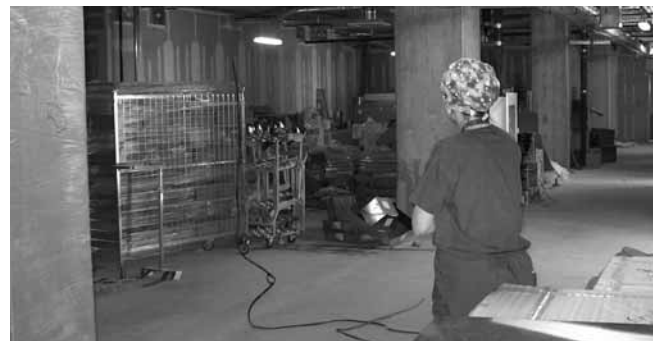
"Shelled-in" space for future development in the OR suite area
